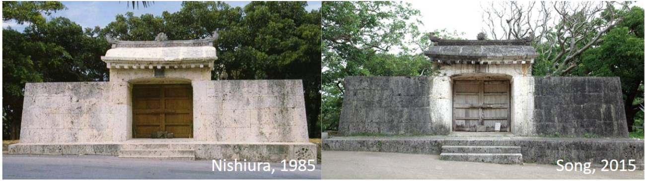
Fig. 1. After completing conservation restoration work of Sonohyan-utaki Ishimon (left) and situation of thirty years later (right).
