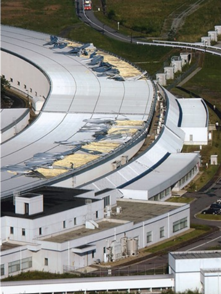
Damage to steel roof sheets due to Typhoon (2004, RIKEN)
