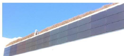
Fig.4 Low reflectance PV modules
