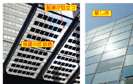
Fig.2 Problems for external wall surface application
